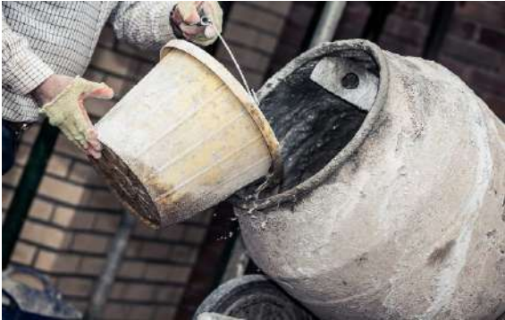
Figure 4: Mixing with a mixer
