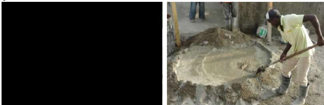
Figure 3: Manual concrete mixing
