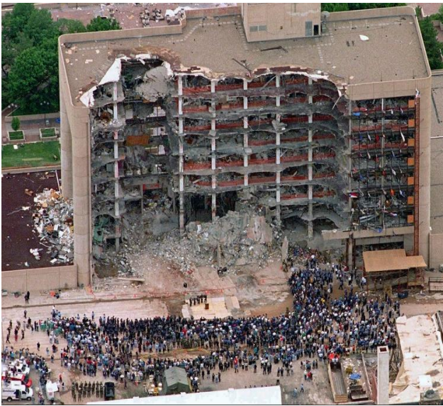
Fig. 1.3 Top view of damaged federal building. (Civil Engineering)
