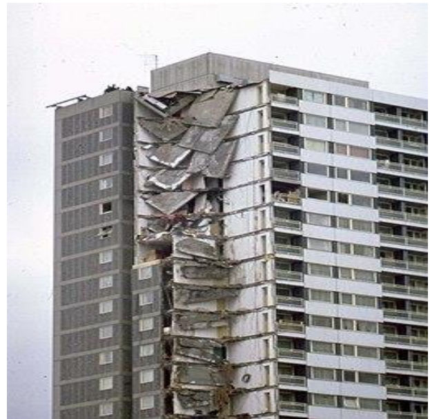
Fig. 1.1 The collapse of one corner of the Ronan building (Wikipedia)
