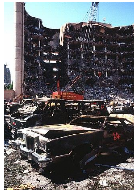
Fig. 1.2 One-third of the Murrah Federal Office damaged. (Wikipedia)
